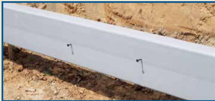
**TIP:** To make sure lineals stay tight against the footing after the concrete pour and prior to backfilling, drywall screws can be used as anchors. Simply screw them partially into the inner (unslotted) surface of the lineals at regular intervals prior to the concrete pour.
